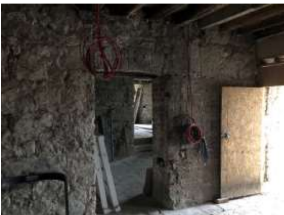
Photo 73 – Room G8 – Brick infill to original arched entrance.
