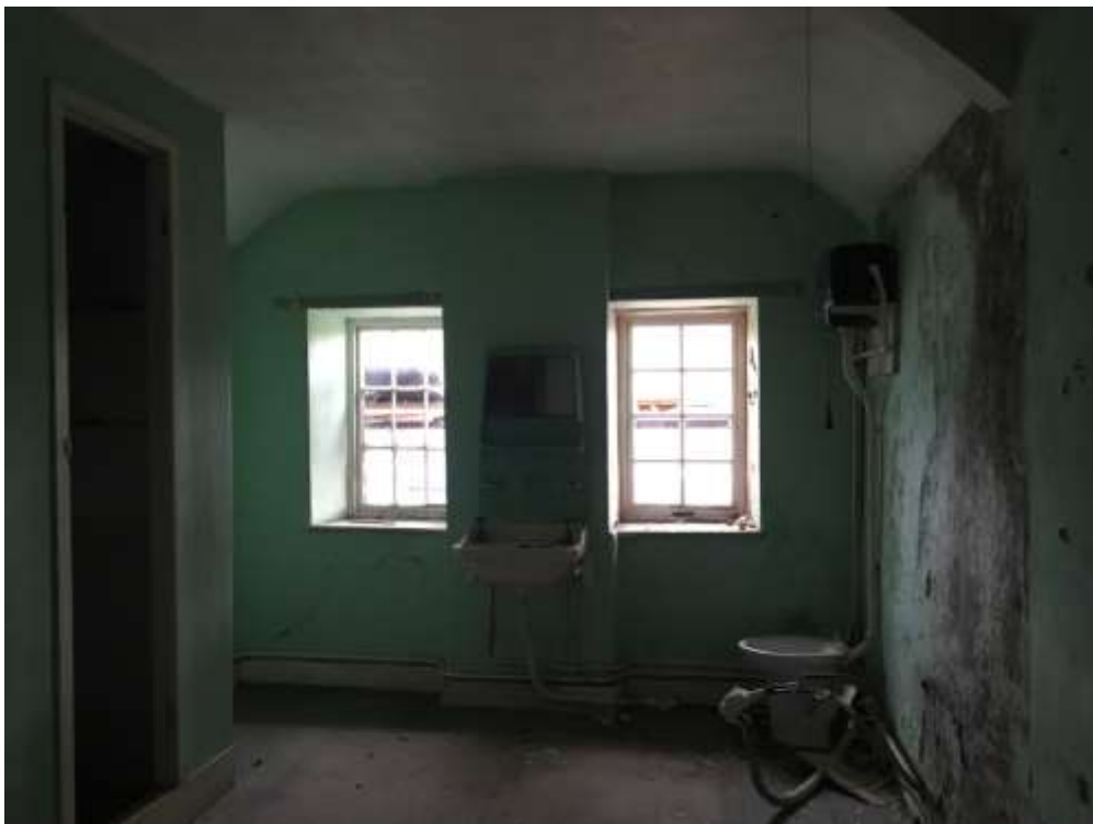
Image F4 (1) – First floor -Room F4
