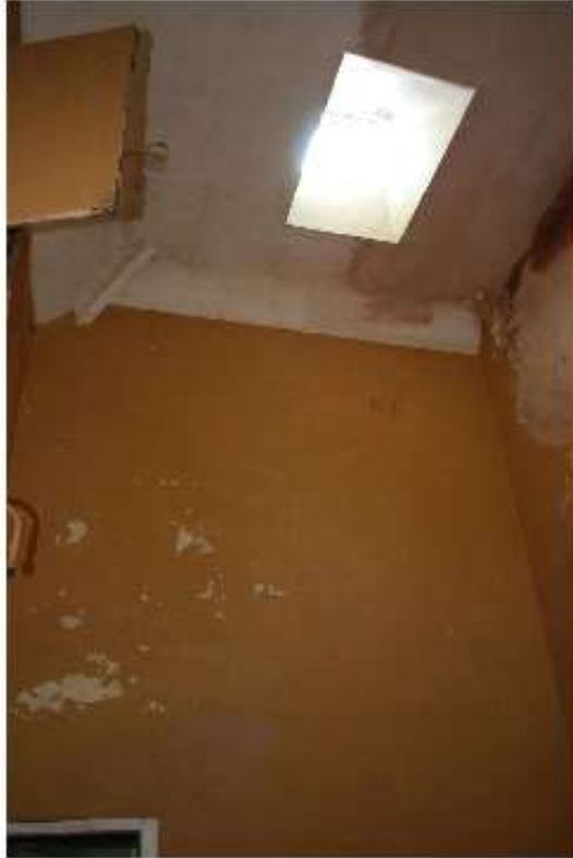
Figure 1.2 Photographs of rooflight – internal
