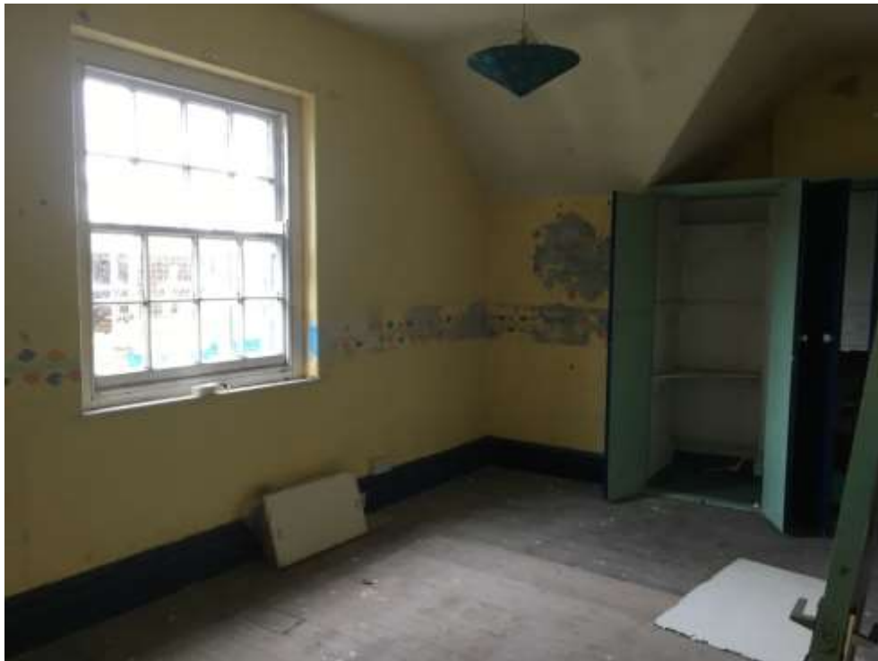
Image F7 (1) – First floor -Room F7
