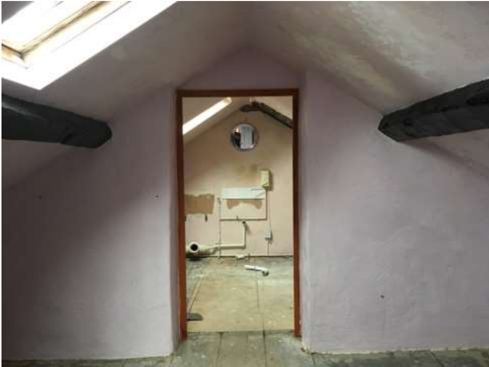
Image F16 (1) – First floor -Room F16
