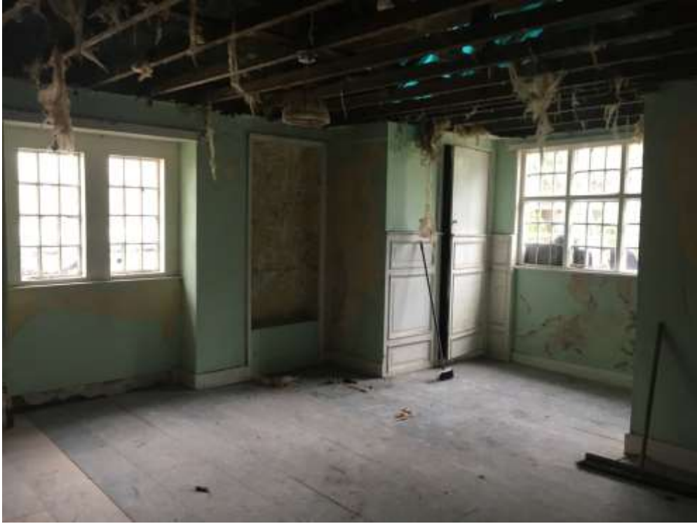
Image F3 (4) – First floor -Room F3
