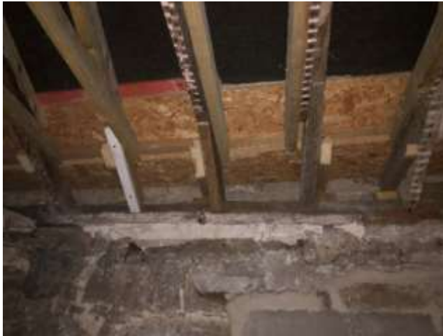
Photo 61 - Room G4 – Replacement of rotten timber box gutter.
