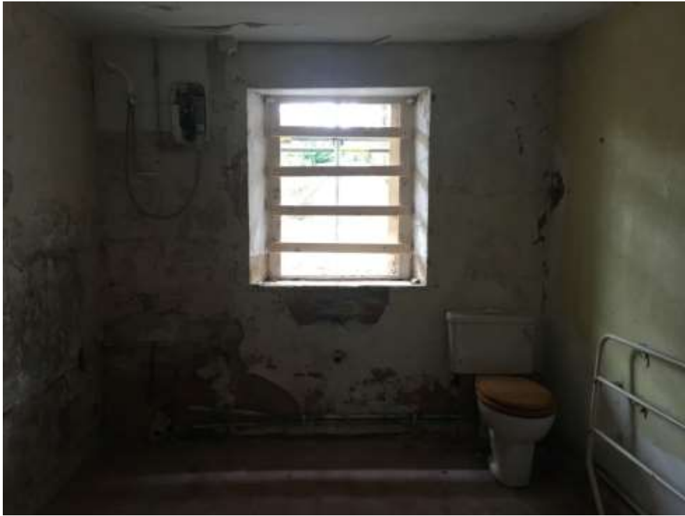
Image G15 (1) - Ground floor -Room G15
