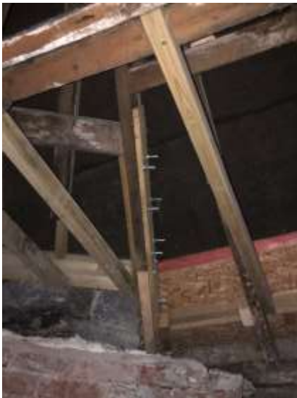
Photos 62 & 63 - Room G4 - Splicing, bracing and replacement of rotten roof and ceiling timbers.
