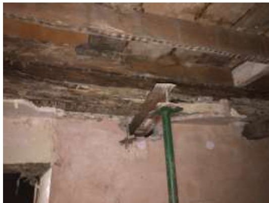
Photos 45 & 46 – Room G2 – Dry rot to main supporting timber beam with temporary support inserted.
