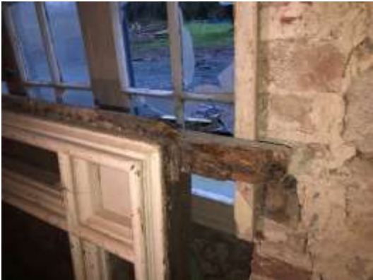
Photos 69 & 70 - Room G11 – Rot to frame of roof light requiring removal to enable repairs to be carried out.
