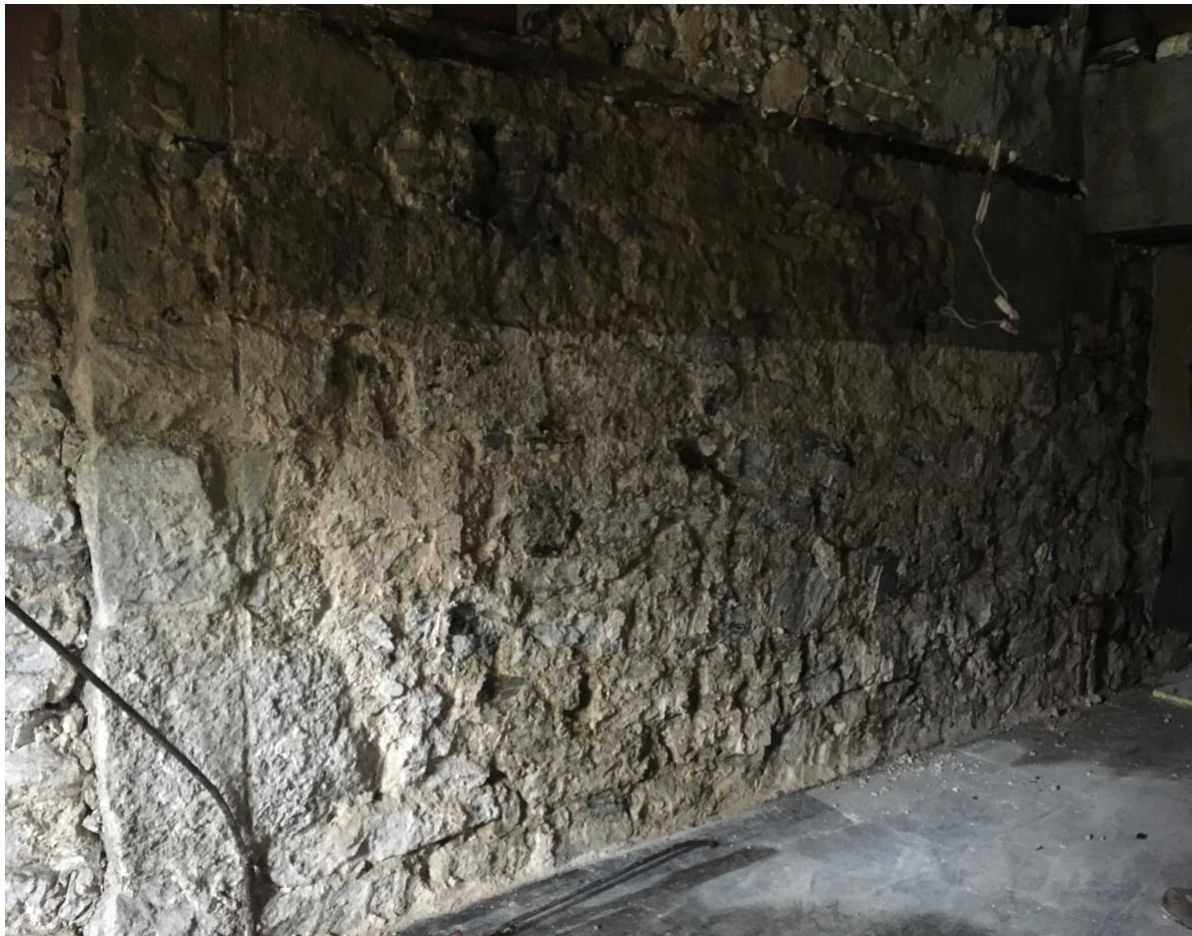
Figure 2: Section of possibly primary (pre-c1830?) wall, room F6.
