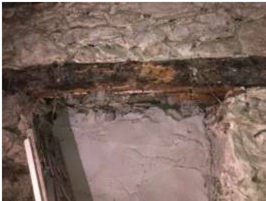
Photos 43 & 44 - Room G2 – Dry rot within lintel and paneling to niche feature.
