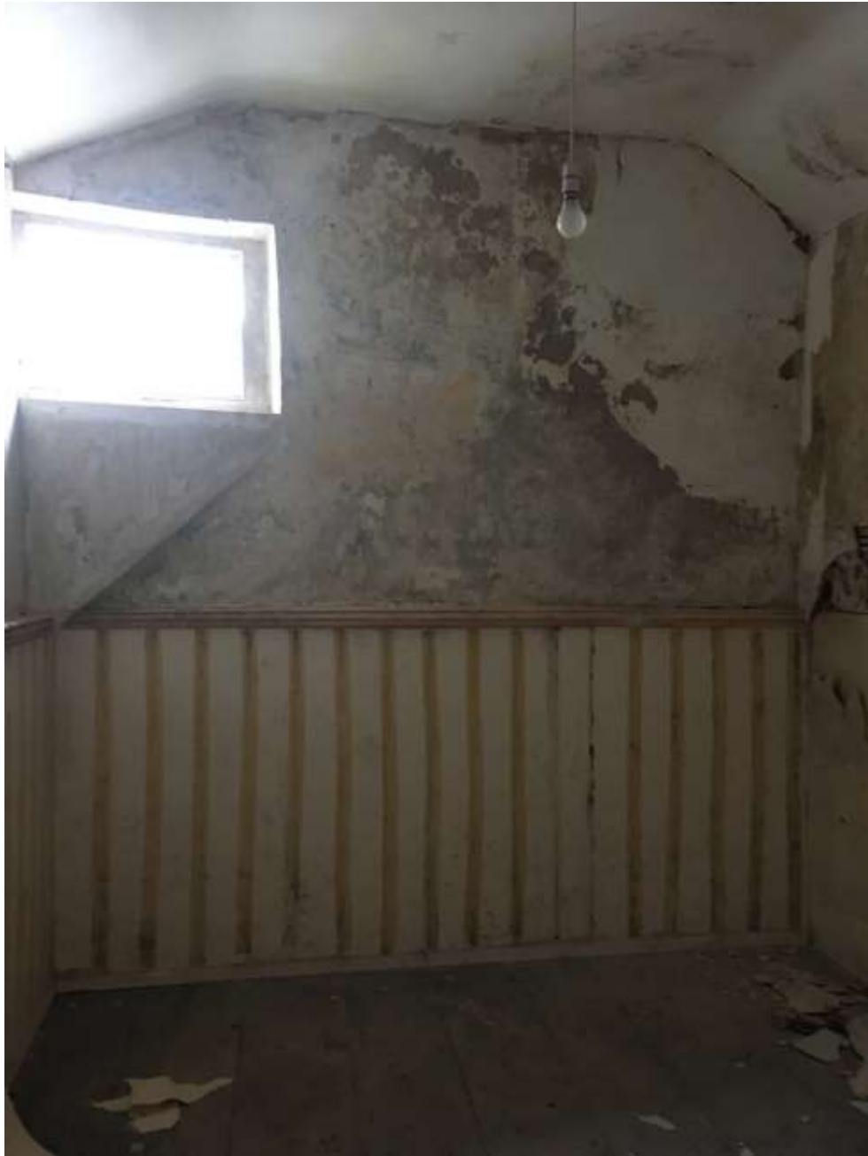
Image F13 (1) – First floor -Room F13
