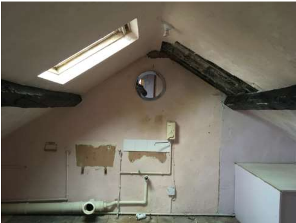
Image F15 (1) – First floor -Room F15
