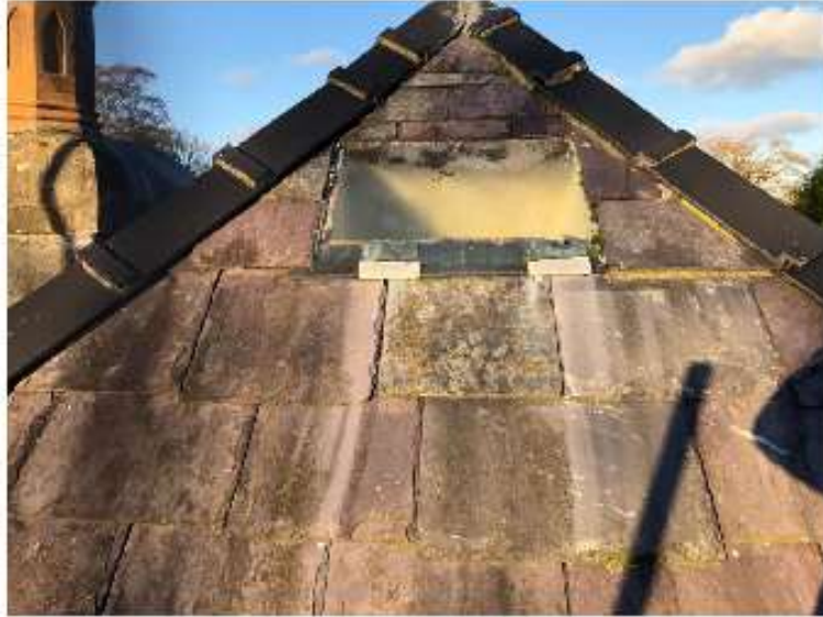
Figure 1.1 Photographs of rooflight - external
