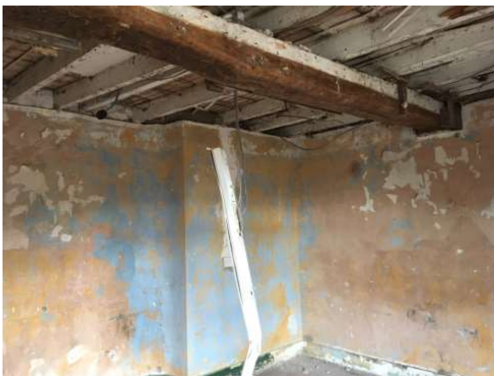
Image G14 (2) - Ground floor -Room G14
