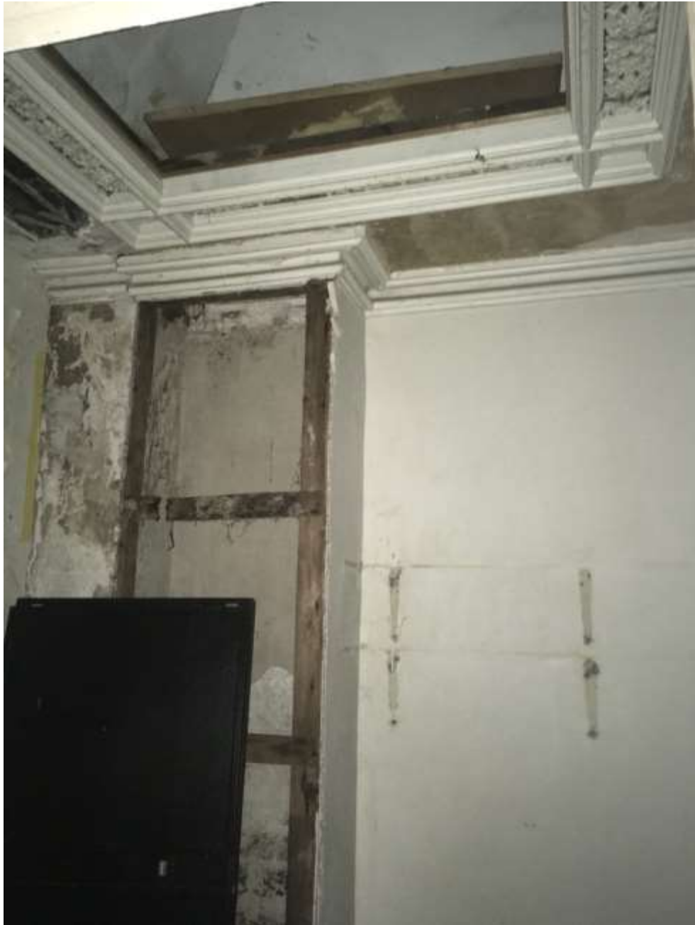
Image G10 (3) - Ground floor -Room G10
