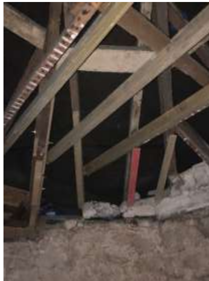
Photos 62 & 63 - Room G4 - Splicing, bracing and replacement of rotten roof and ceiling timbers.
