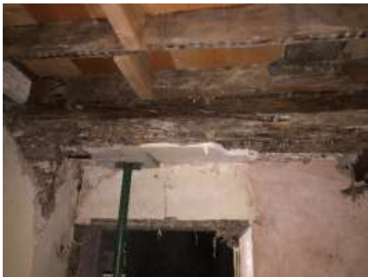
Photos 45 & 46 – Room G2 – Dry rot to main supporting timber beam with temporary support inserted.
