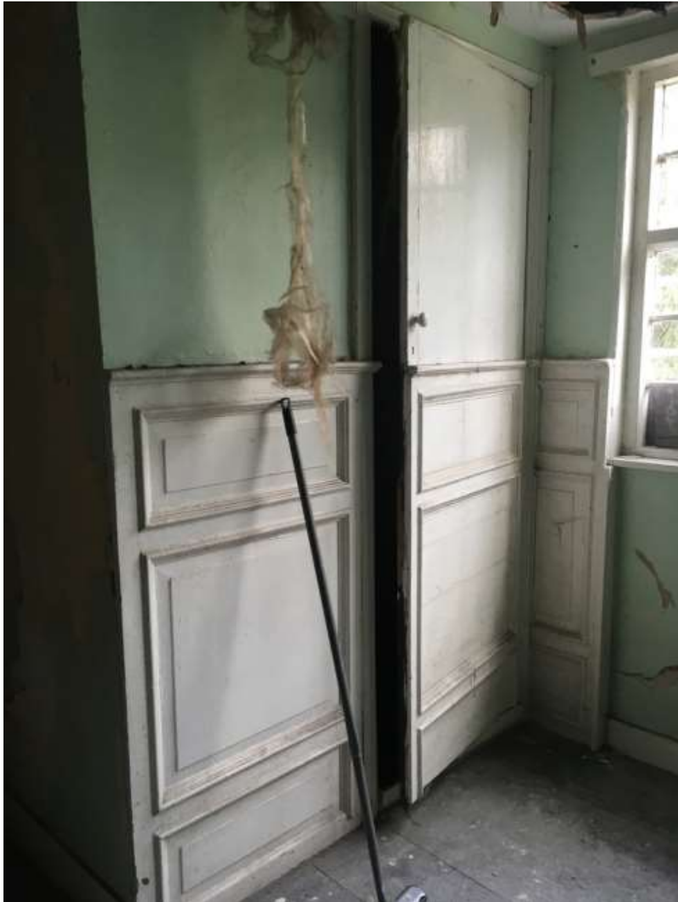
Image F3 (1) – First floor -Room F3
