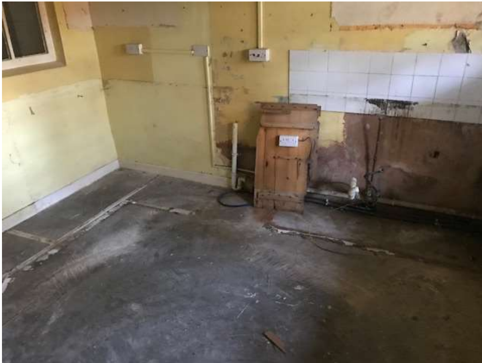
Image G13 (1) - Ground floor -Room G13
