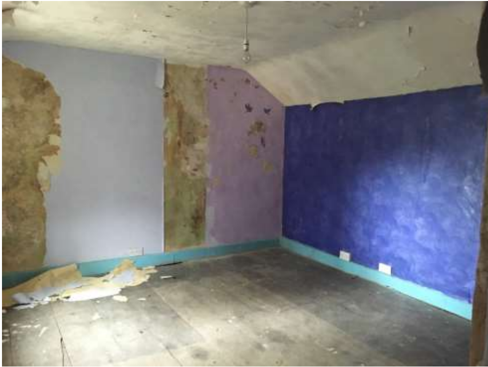
Image F14 (1) – First floor -Room F14
