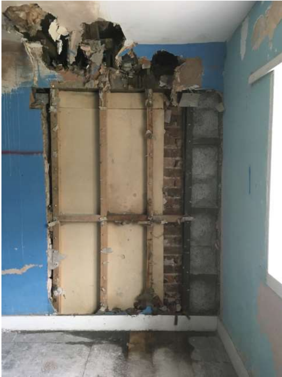
Image F2 (2) – First floor -Room F2
