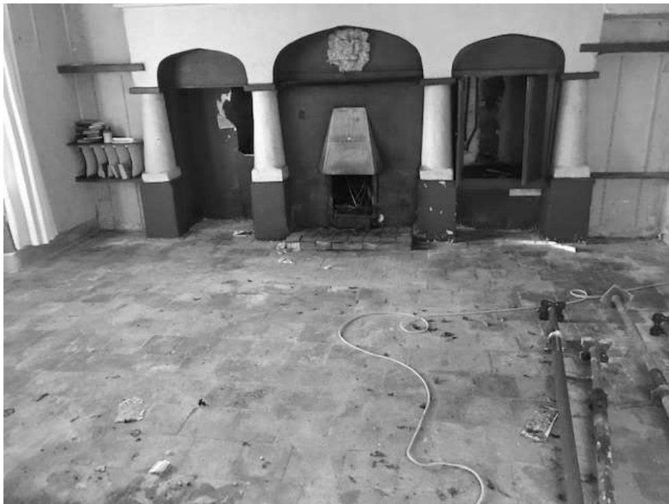
Image G8 (2) - Ground floor -Room G8
