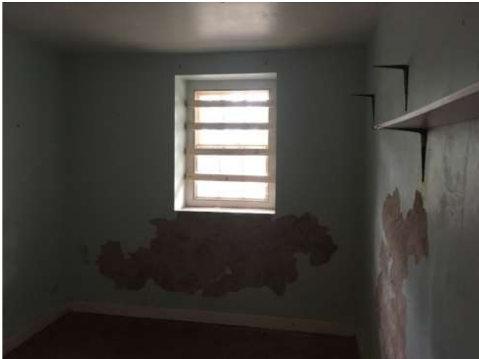
Image G16 (1) - Ground floor -Room G16
