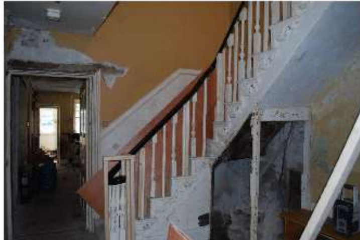
Figure 1.3 Photograph of staircase in tower
