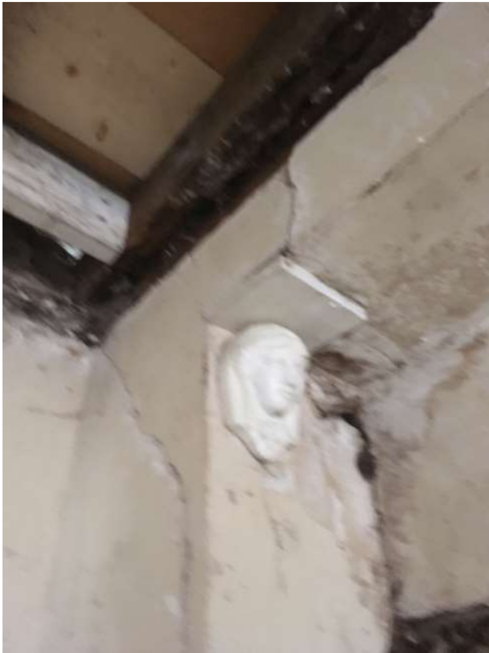
Image G2 (5) - Ground floor -Room G2
