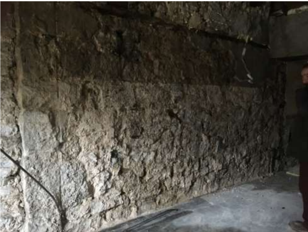
Image F6 (2) – First floor -Room F6
