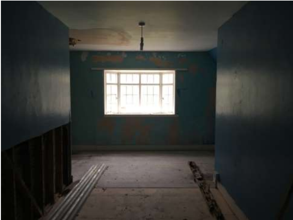
Image F2 (1) – First floor -Room F2
