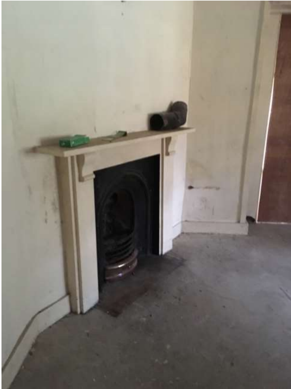
Image G3 (2) - Ground floor -Room G3
