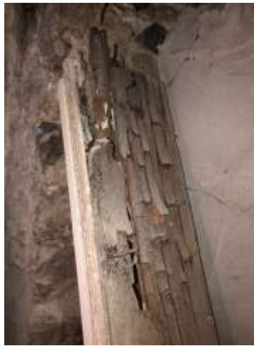
Photos 43 & 44 - Room G2 – Dry rot within lintel and paneling to niche feature.
