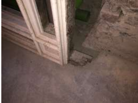
Photos 69 & 70 - Room G11 – Rot to frame of roof light requiring removal to enable repairs to be carried out.
