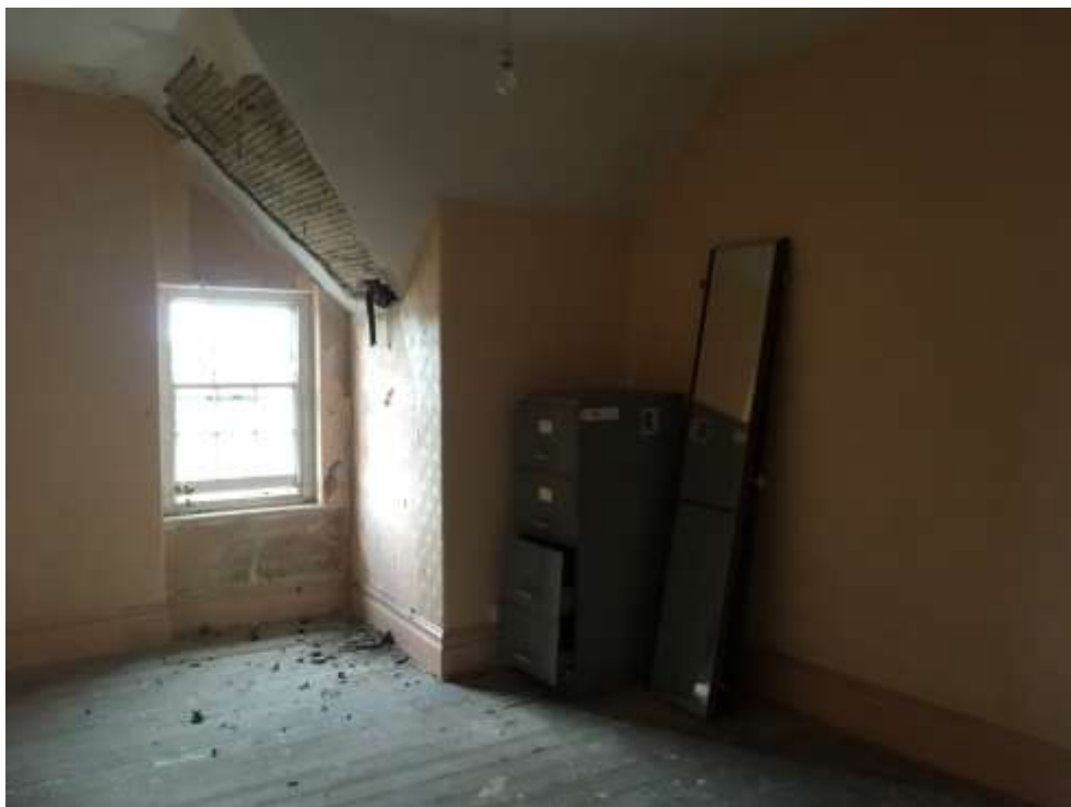
Image F8 (1) – First floor -Room F8
