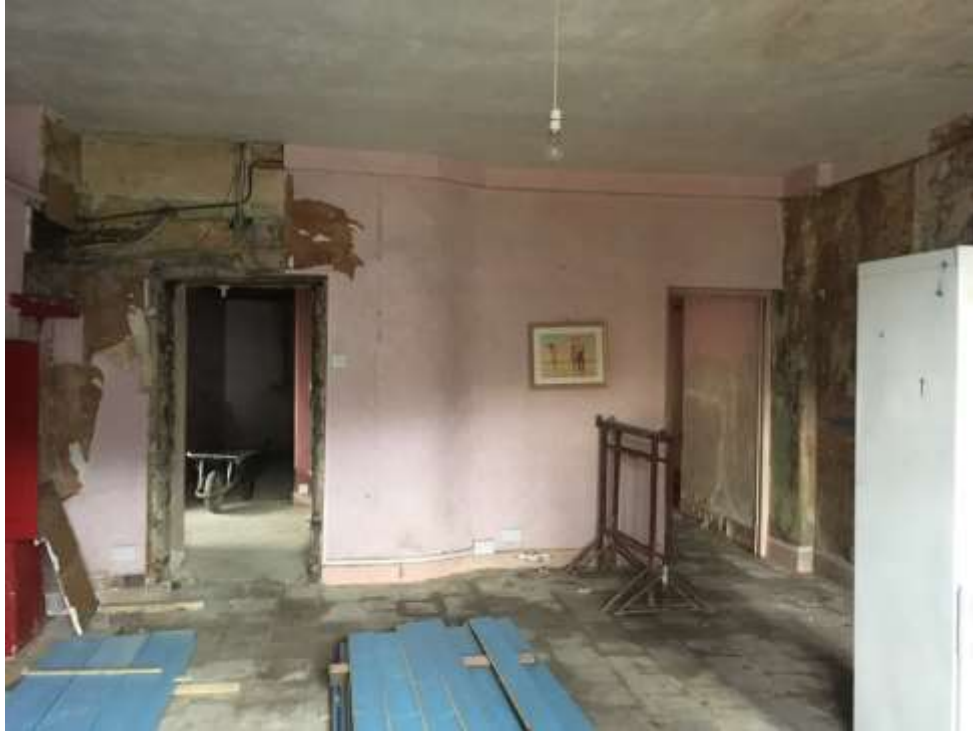
Image G8 (1) - Ground floor -Room G8
