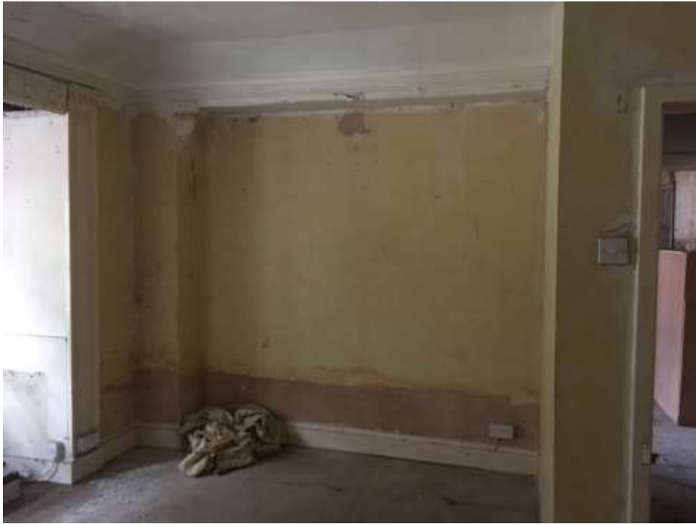
Image G3 (3) - Ground floor -Room G3
