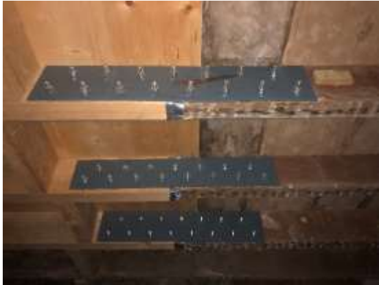
Photos 41 & 42 - Room G2 – Previous repairs to floor joists and evidence of dry rot effecting these replacement timbers.
