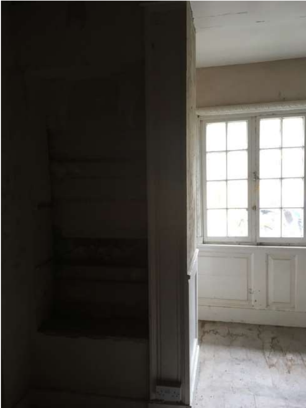
Image G2 (3) - Ground floor -Room G2
