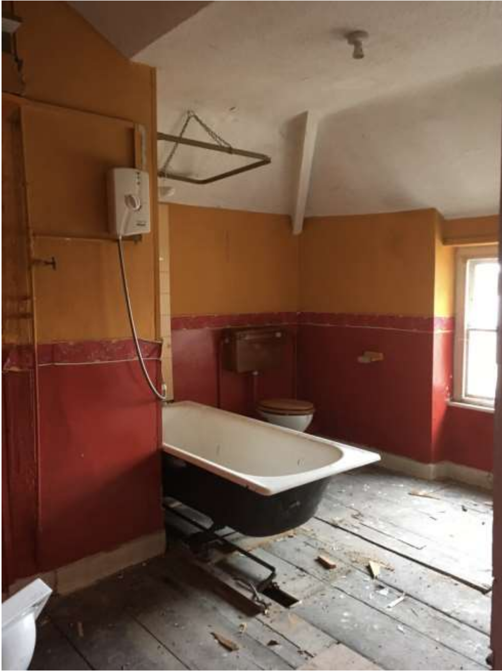
Image F11 (1) – First floor -Room F11
