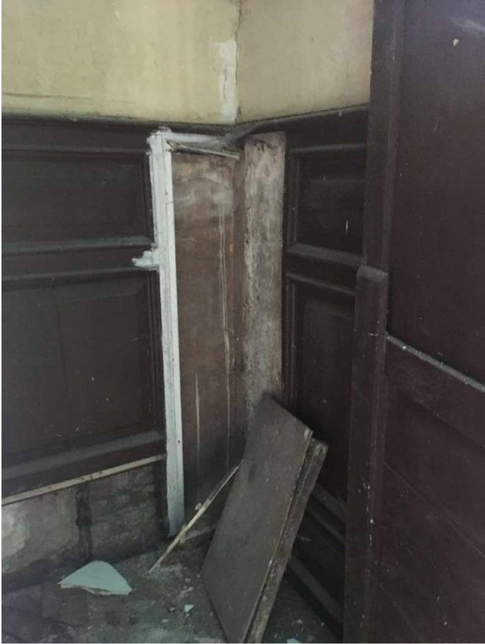
Image F3 (3) – First floor -Room F3
