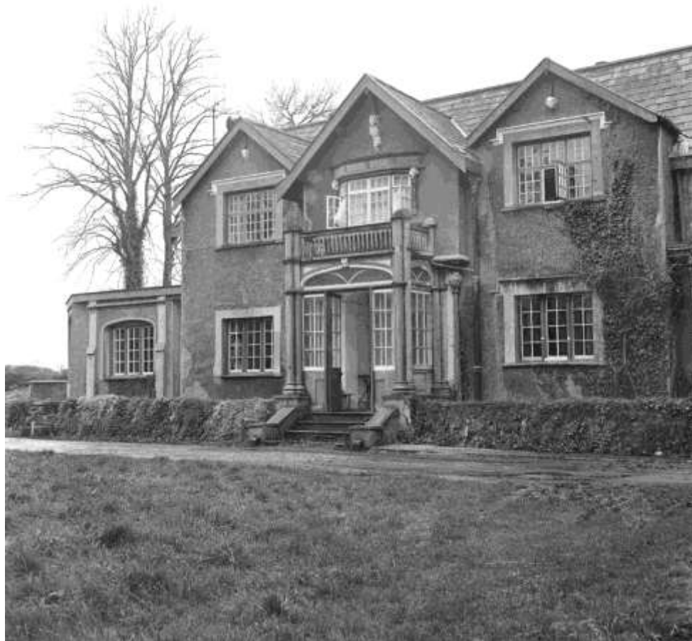
Image SE (6) – South West Elevation – Late 20 th Century Showing Porch
