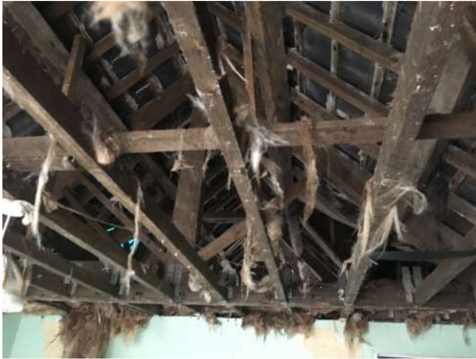
Image F2 (3) – First floor -Room F2
