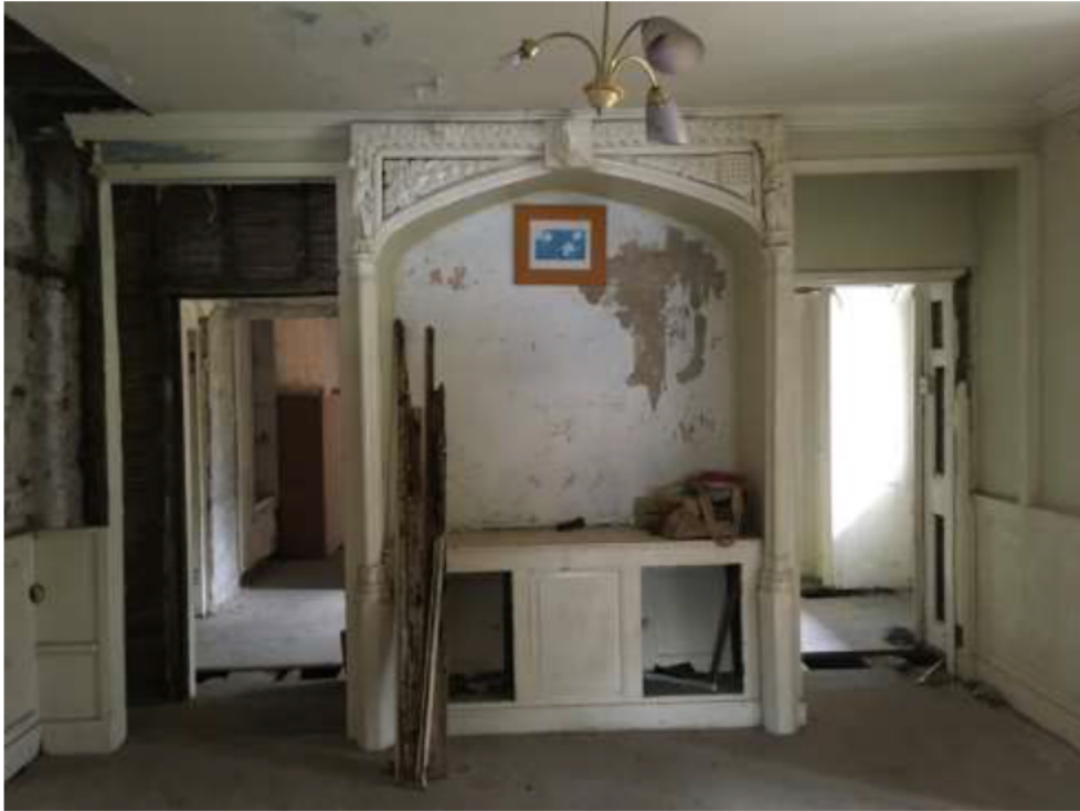
Image G1 (7) - Ground floor -Room G1
