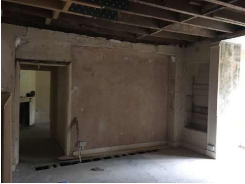
Image G2 (4) - Ground floor -Room G2
