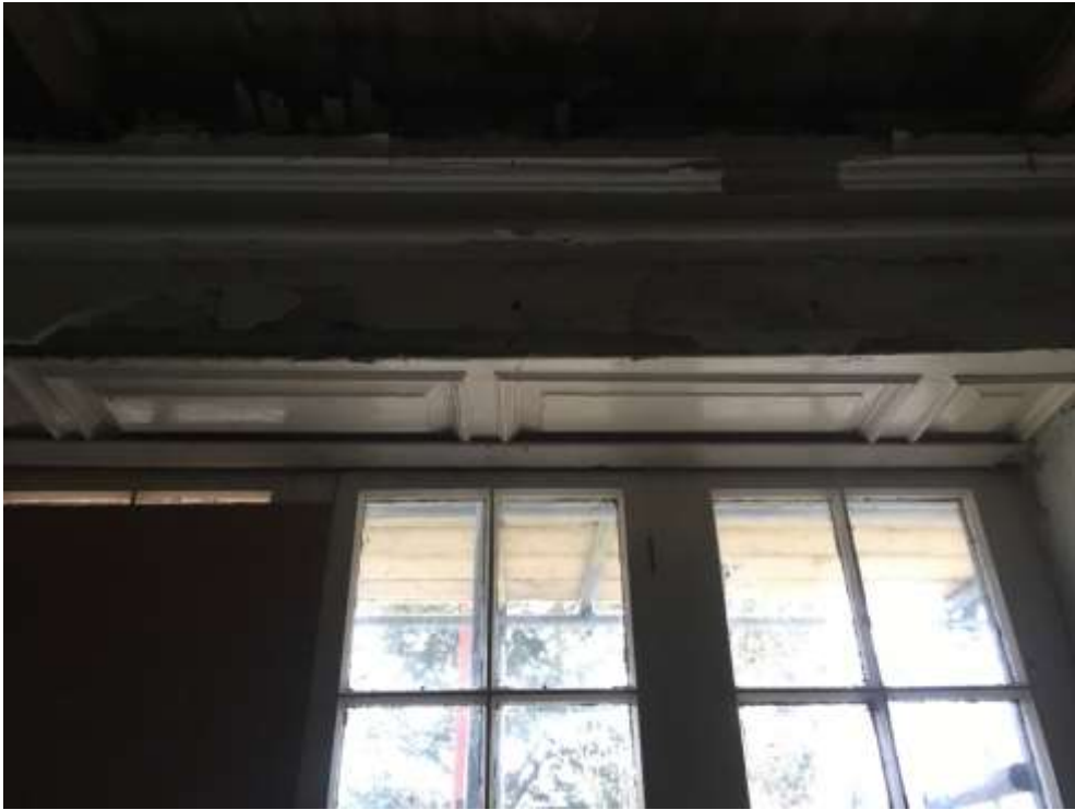
Image G7 (1) - Ground floor -Room G7
