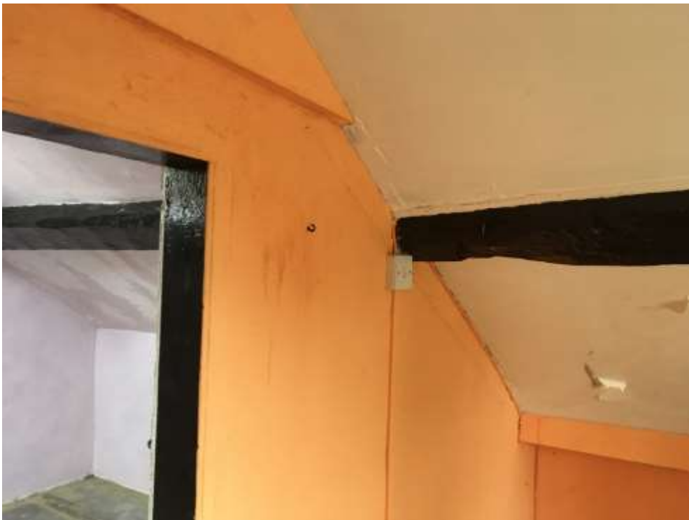
Image F17 (1) – First floor -Room F17
