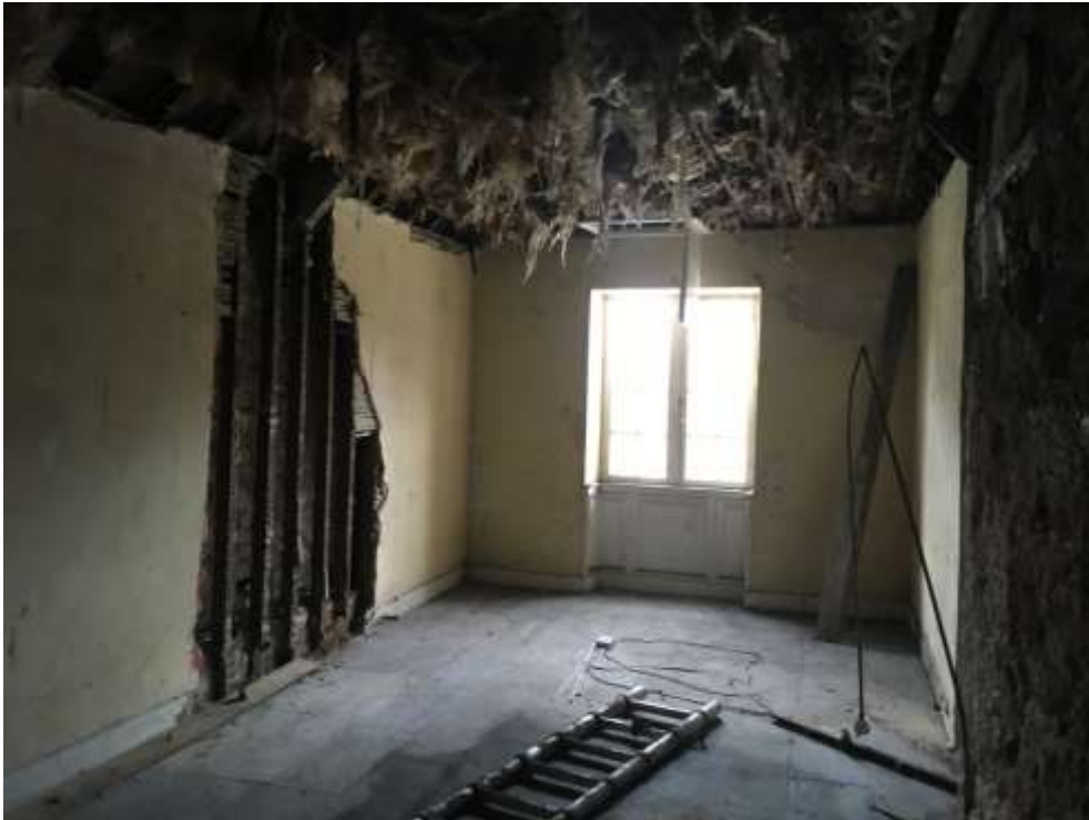
Image F6 (1) – First floor -Room F6
