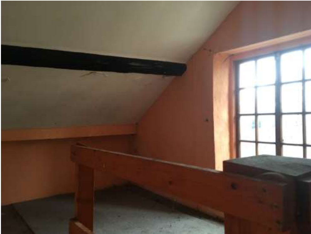
Image F17 (2) – First floor -Room F17
