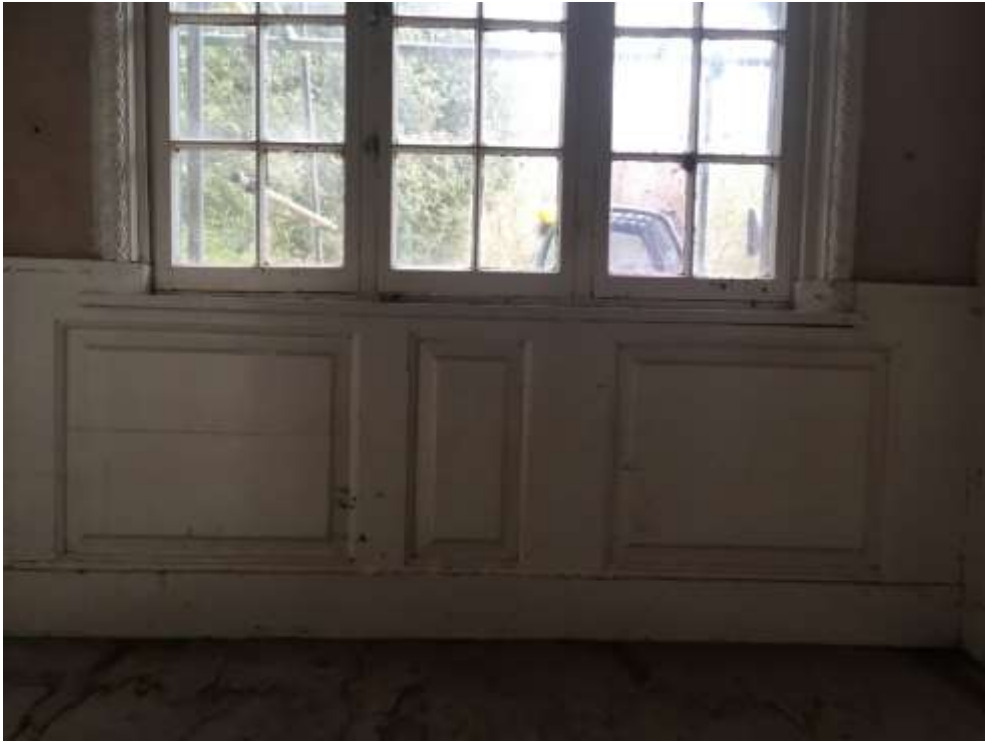
Image G2 (2) - Ground floor -Room G2
