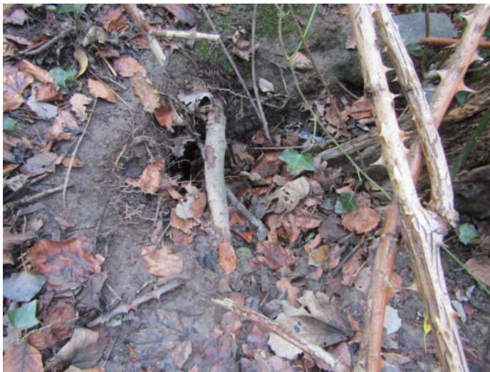
Photo 14: Tunnel entrance in woodland blocked by fallen leaves (Jan 2022).
