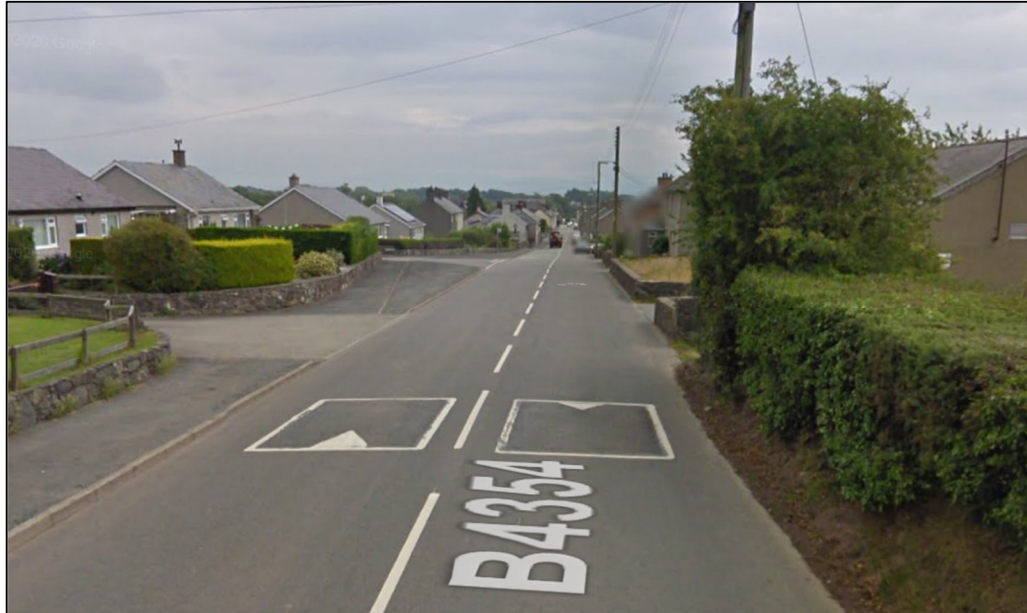
Figure 2.4 – Speed Cushions on the B4354
